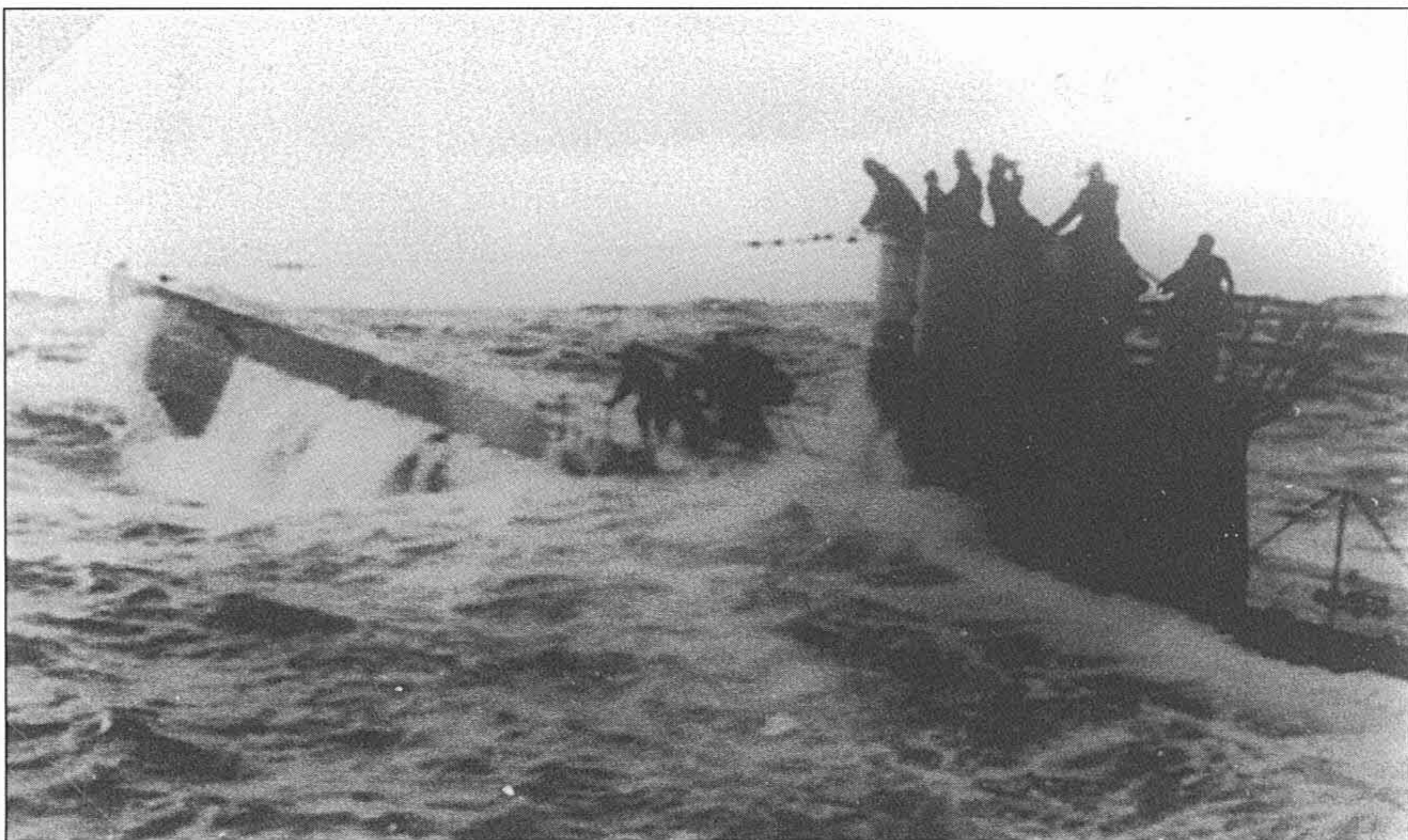
This action photograph, taken during a war patrol, shows U-130, a Type IXC, in heavy seas. One can easily imagine the difficulty the gun crew would have had in keeping their footing on the heaving deck. Note the seawater pouring from the vents leading to the free-flooding area between the outer casing and pressure hull.
